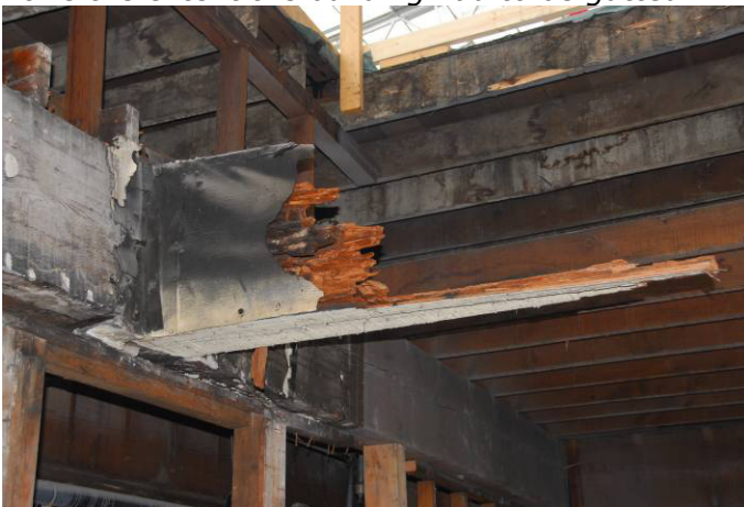
Examples of rotten beams. Beams have been or will be replaced on every level in the building.
