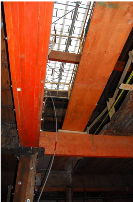
New beams installed.
