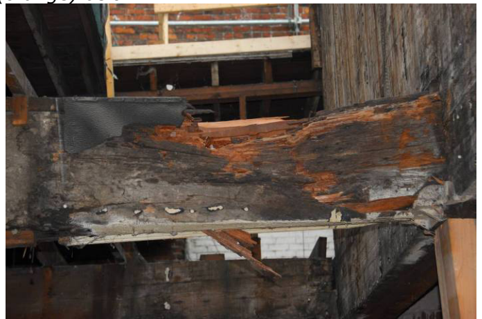
Examples of rotten beams. Beams have been or will be replaced on every level in the building.
