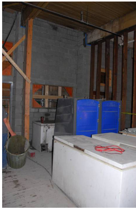
The back wall was structurally unsound and has been replaced.
