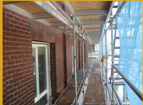
Repointed brick work.
