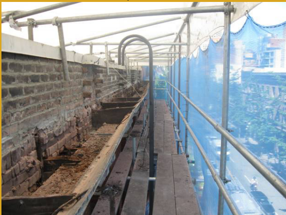
Demolition of the sheet metal cornice.
