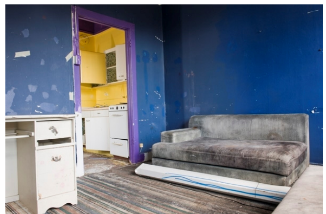
Park Hotel: a typical unit pre-renovations
